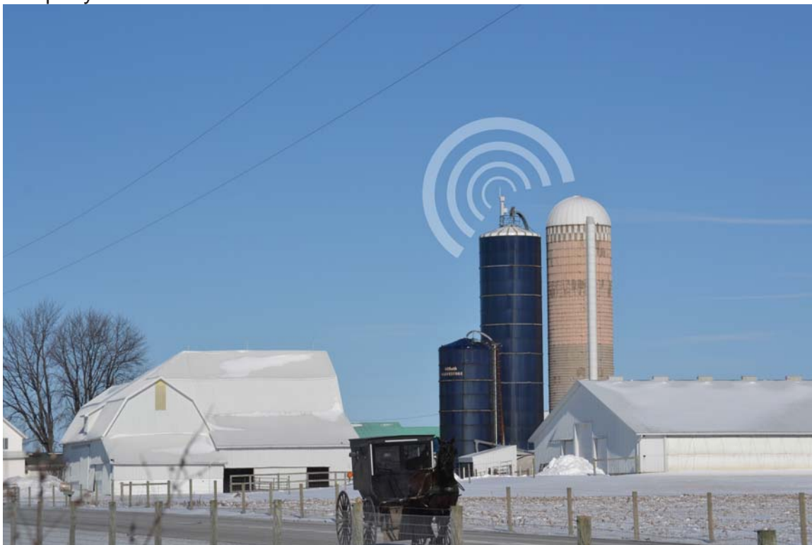
Figure 2: Wireless broadband antenna atop a silo on an Amish farm
